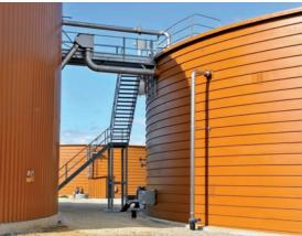
A catwalk, accessible via a stairway, connects the LIPP KomBio-Reactor with the LIPP Post-Digester
