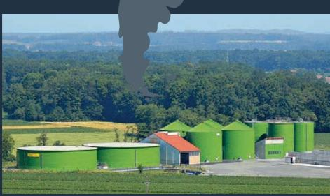
Biogas plant in Austria, capacity approx 1 MWel Total input p.a.: 21.900 t liquid manure, glycerine, silage maize, grain maize
