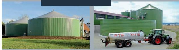
torage tank for fermented substrate with membrane cover
