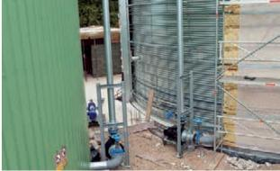
Assembly of wall heating, insulation, and outer cladding
