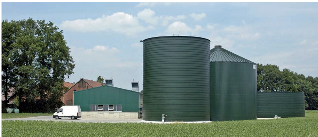
Biogas plant in Germany with a LIPP-BETAVATOR.
