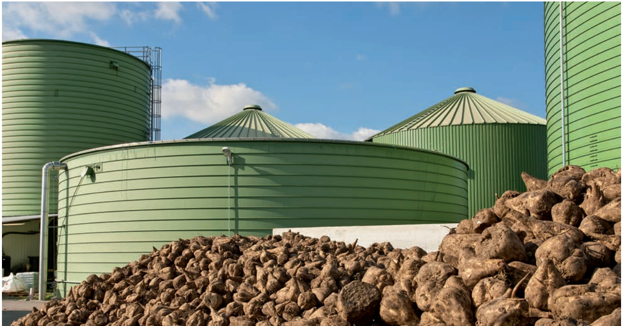
Biogas plant in Germany using sugar beet as the only substrate. The heat is utilized by an adjoining industrial estate.
