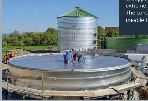
Assembly of stainless steel membrane cover
