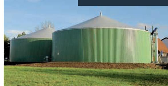
Storage tank for fermented substrate with membrane cover
