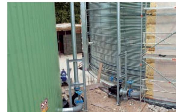
Assembly of wall heating, insulation, and outer cladding
