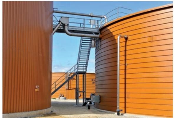
A catwalk, accessible via a stairway, connects the LIPP KomBio-Reactor with the LIPP Post-Digester
