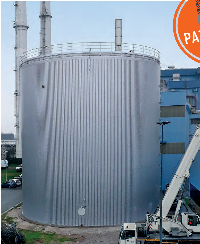
LIPP Gross-Pufferspeicher, 5.200 m 3 Volumen
