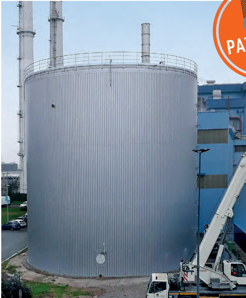
LIPP Gross-Pufferspeicher, 5.200 m 3 Volumen
