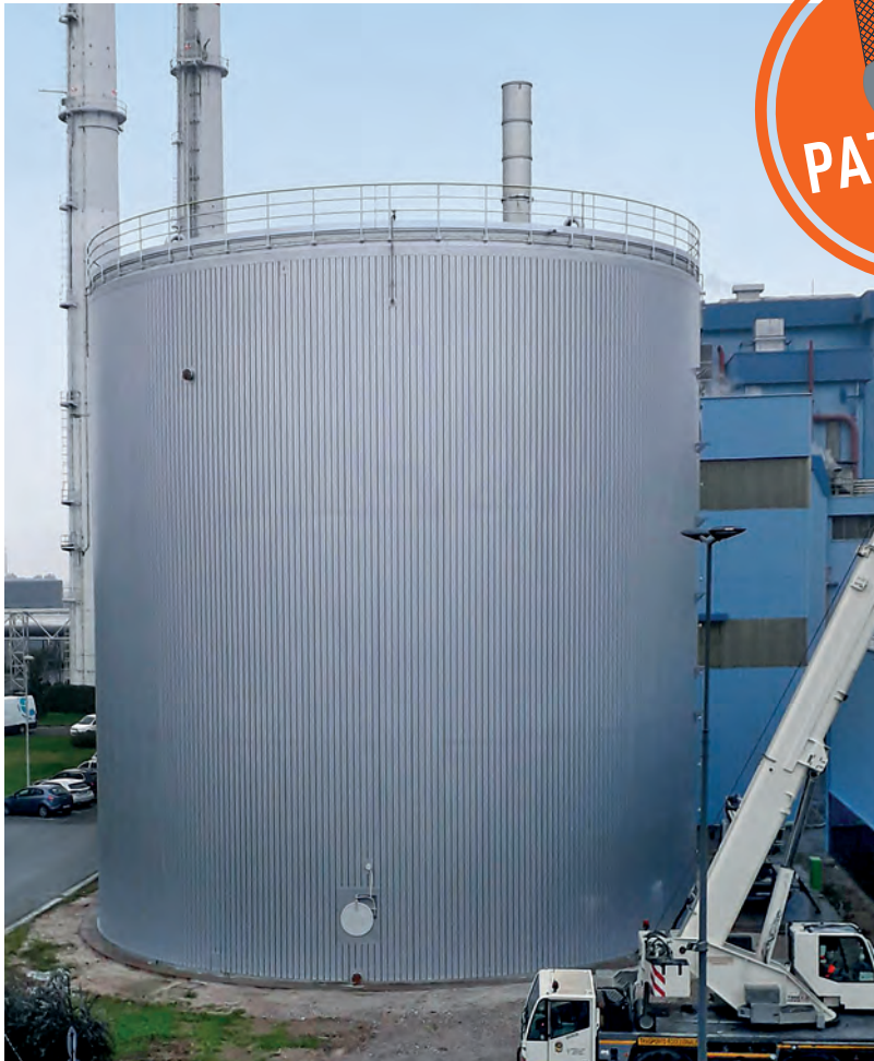
LIPP Gross-Pufferspeicher, 5.200 m 3 Volumen
