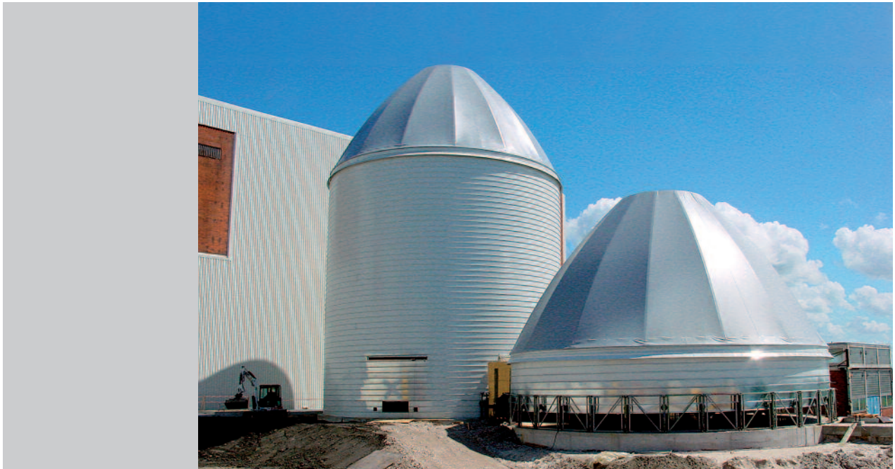
Electricity plant in Germany: LIPP Bulk Storage Silos for storage of woodchips
