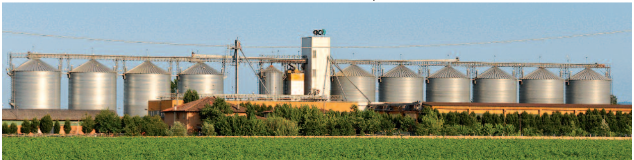
Agricultural Cooperative in Italy: LIPP Bulk Storage Silos for grain storage
