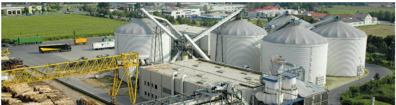
Wood chips plant in Germany: LIPP Bulk Storage Silos for the storage of woodchips
