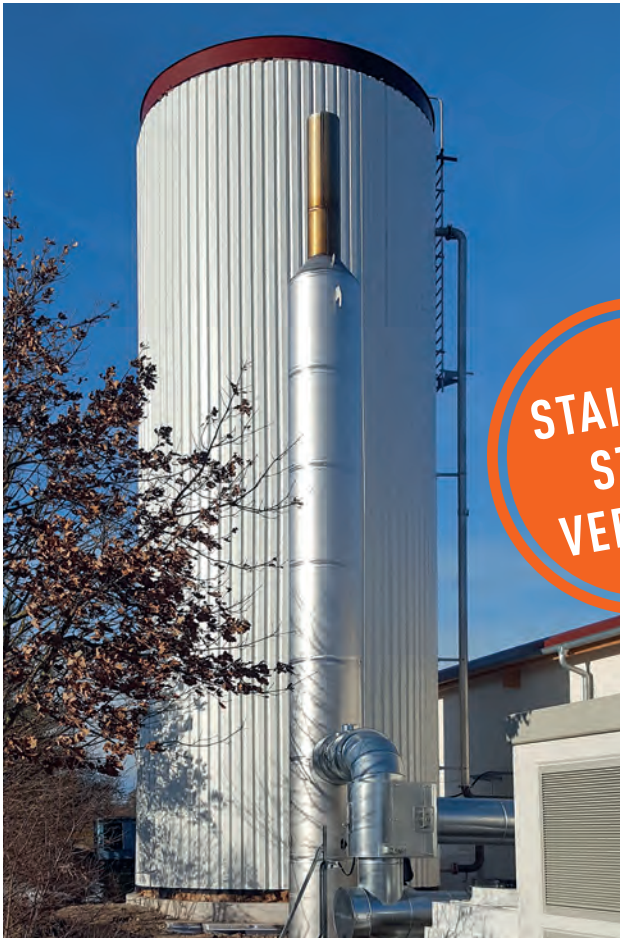
LIPP Thermal Storage Tank, 300 m 3 volume
