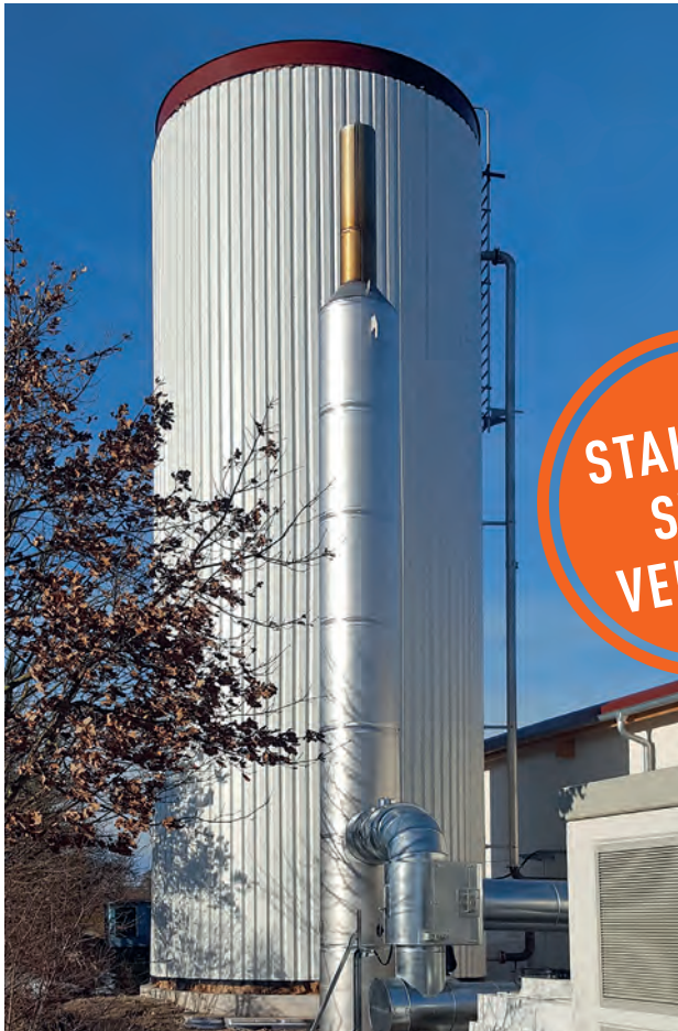
LIPP Thermal Storage Tank, 300 m 3 volume
