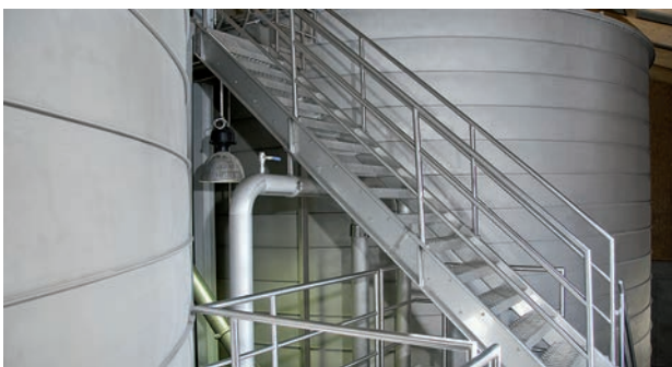
LIPP stainless steel container serving as drinking water tank, welded
