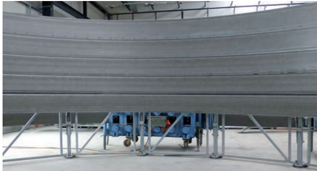
Interior view, LIPP steel container during production
