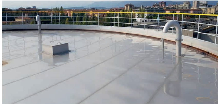
Figure 3. The stainless-steel membrane cover is a self-supporting, lightweight construction with high mechanical strength that can withstand snow loads and strong winds. It is prefabricated in the factory, transported to the construction site, and installed on site
