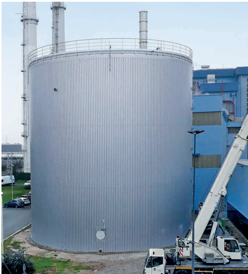
Figure 2. The project "Lamarmora" after completion
